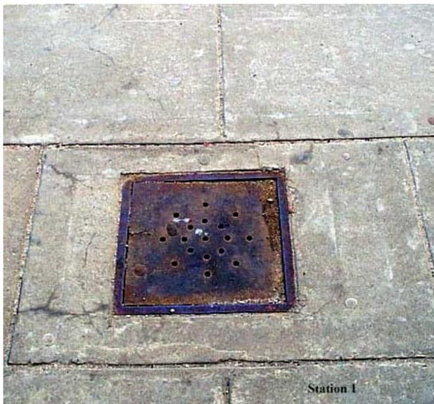
Close up of catch basin at bottom of picture on right. In picture on right the catch basin are in a row and transfer surface water to the storm sewer below the surface.
