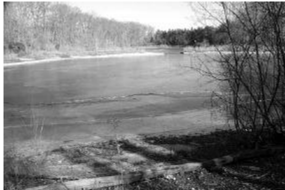
Standing water recharge basin
